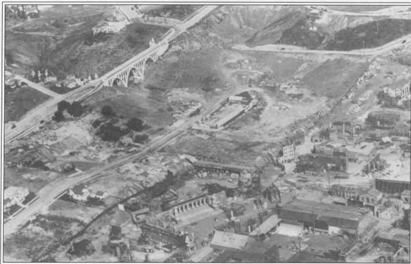
Franklin Hill in 1928, after Contractor Metcalf has done his work
